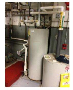
Gas-fired water heater (left) and electric water heater (right)
