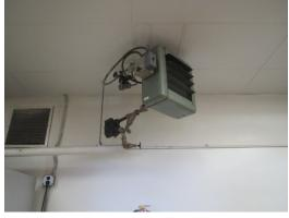
T-static Steam Trap on the Unit Heater
