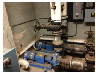
Heating hot water pumps for 1967 section of building
