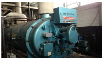
Fire tube heating hot water boiler
