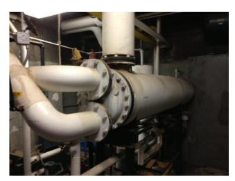
Steam to heating hot water heat exchanger (1 of 2)
