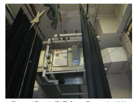
Float and T-static (F&T) Steam Trap on the AHU
