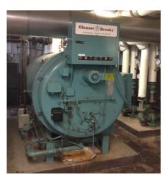
Fire tube heating hot water boiler
