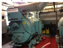
Fire tube hot water boiler
